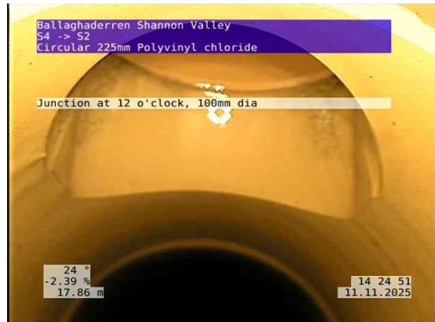
4, 00:02:19, 17.86 m Junction at 12 o'clock, 100mm dia
