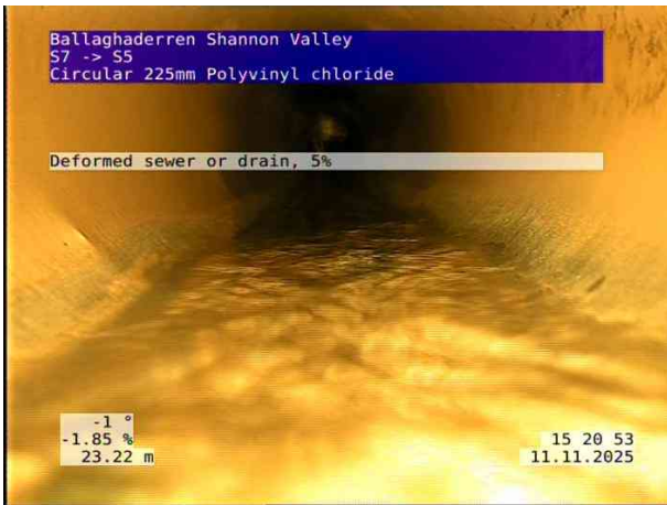
5, 00:02:48, 23.22 m Deformed sewer or drain, 5%
