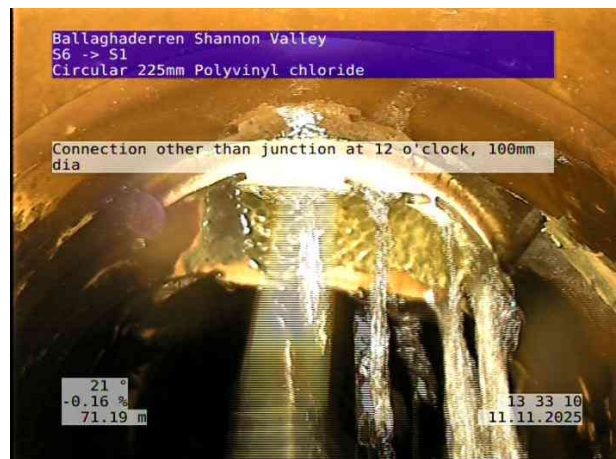
4, 00:06:57, 71.19 m Connection other than junction at 12 o'clock, 100mm dia
