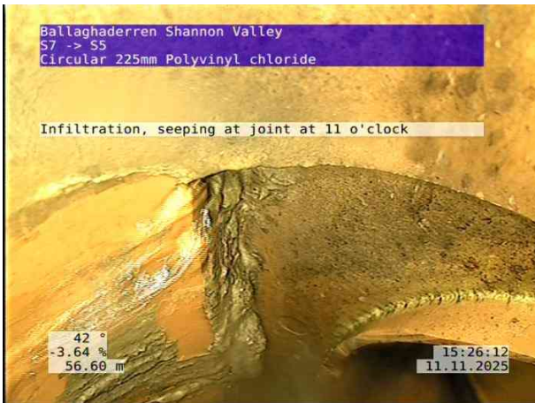
11, 00:06:39, 56.60 m Infiltration, seeping at joint at 11 o'clock
