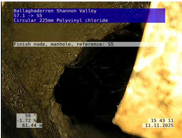
11, 00:07:54, 61.44 m Finish node, manhole, reference: S5
