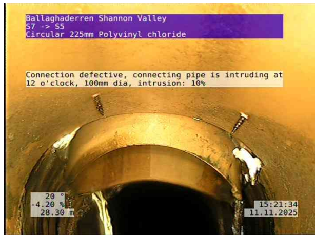
6, 00:03:17, 28.30 m Connection defective, connecting pipe is intruding at 12 o'clock, 100mm dia, intrusion: 10%
