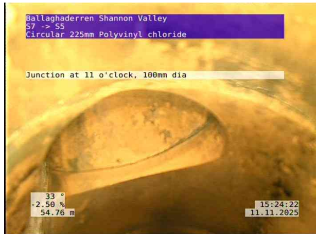
8, 00:05:48, 54.76 m Junction at 11 o'clock, 100mm dia
