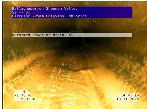
4, 00:02:00, 15.91 m Deformed sewer or drain, 5%
