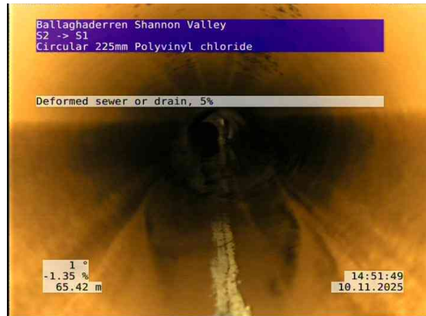
12, 00:11:03, 65.42 m Deformed sewer or drain, 5%
