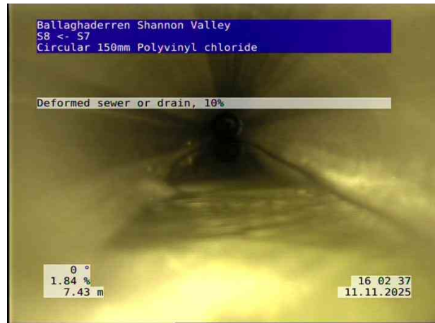
2, 00:01:50, 7.43 m Deformed sewer or drain, 10%
