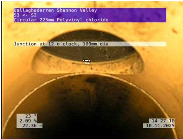
5, 00:02:47, 22.36 m Junction at 12 o'clock, 100mm dia
