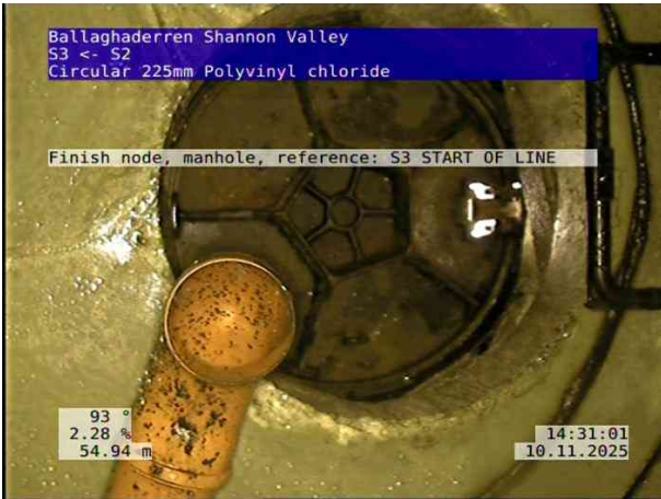
9, 00:06:13, 54.95 m Finish node, manhole, reference: S3, START OF LINE
