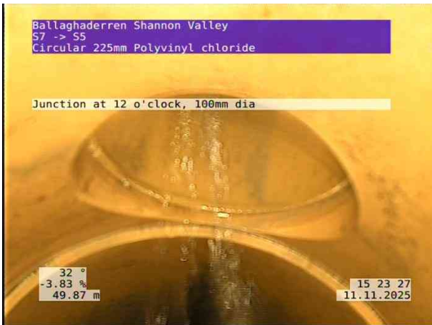
7, 00:05:06, 49.87 m Junction at 12 o'clock, 100mm dia
