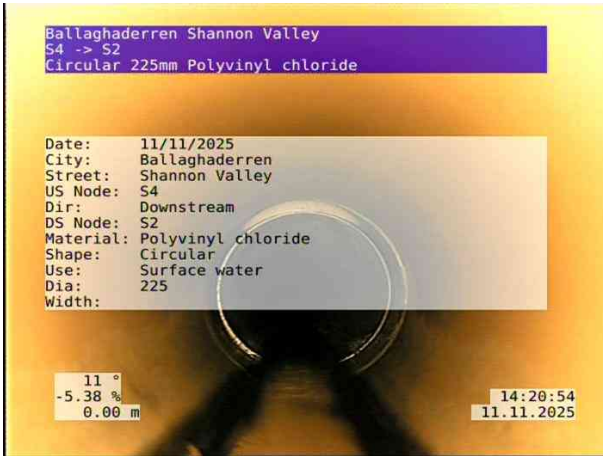
1, 00:00:00, 0.00 m Start node, manhole, reference: S4
