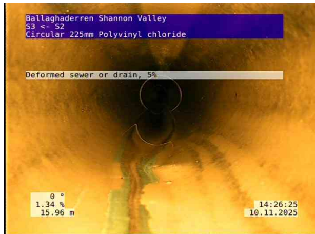
4, 00:02:08, 15.96 m Deformed sewer or drain, 5%
