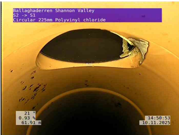
11, 00:10:02, 61.91 m Junction at 12 o'clock, 100mm dia
