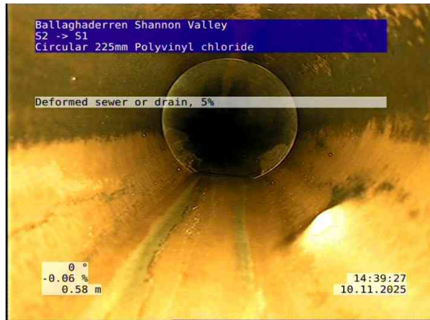
2, 00:00:21, 0.58 m Deformed sewer or drain, 5%
