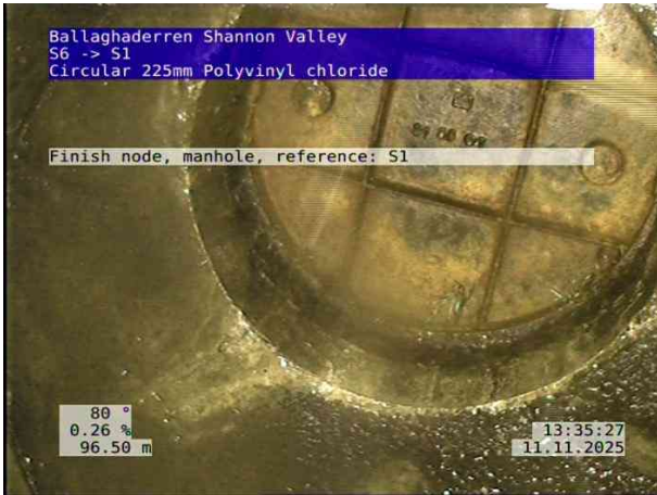
5, 00:09:07, 96.50 m Finish node, manhole, reference: S1
