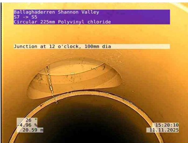
3, 00:02:13, 20.60 m Junction at 12 o'clock, 100mm dia
