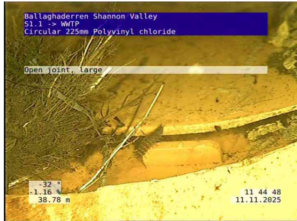
6, 00:10:18, 38.78 m Open joint, large
