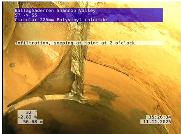
12, 00:06:53, 56.68 m Infiltration, seeping at joint at 2 o'clock
