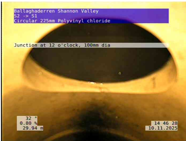
7, 00:06:19, 29.95 m Junction at 12 o'clock, 100mm dia
