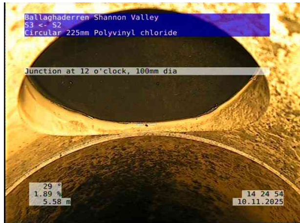
2, 00:00:44, 5.58 m Junction at 12 o'clock, 100mm dia
