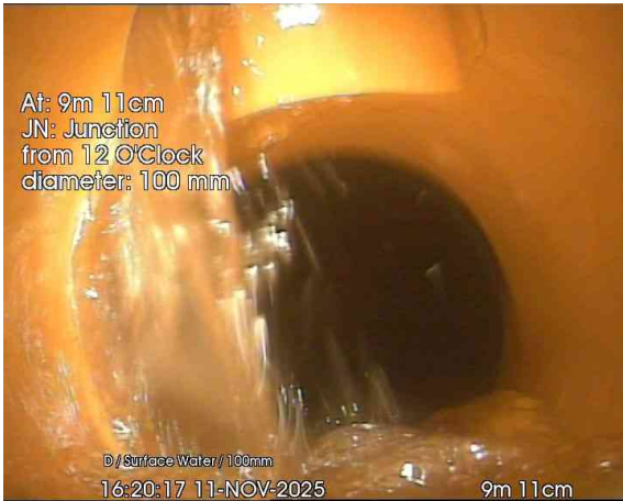
5, 00:00:43, 9.11 m Junction at 12 o'clock, 100mm dia
