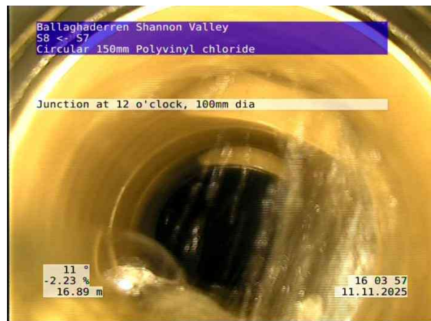
4, 00:03:01, 16.89 m Junction at 12 o'clock, 100mm dia
