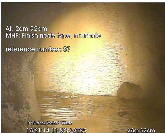
7, 00:01:29, 26.92 m Finish node, manhole, reference: S7
