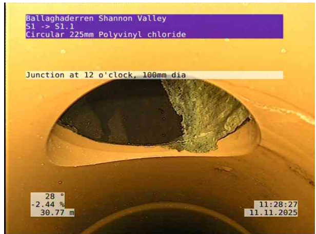
4, 00:03:09, 30.77 m Junction at 12 o'clock, 100mm dia
