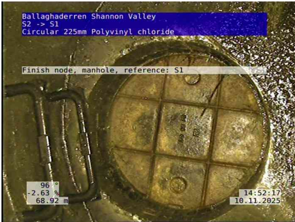
13, 00:11:27, 68.92 m Finish node, manhole, reference: S1
