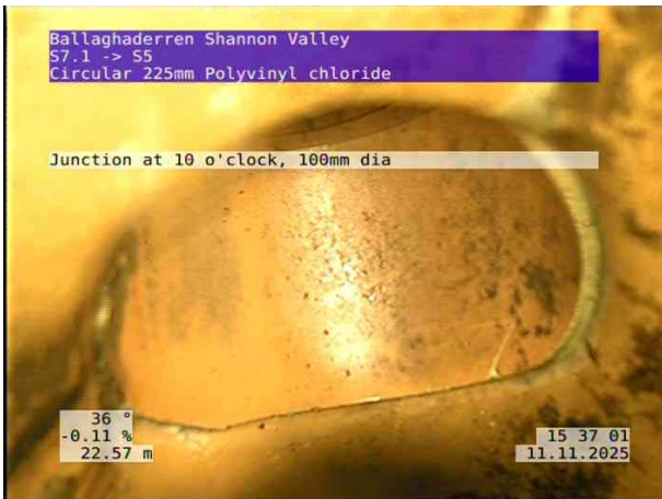
3, 00:03:14, 22.57 m Junction at 10 o'clock, 100mm dia
