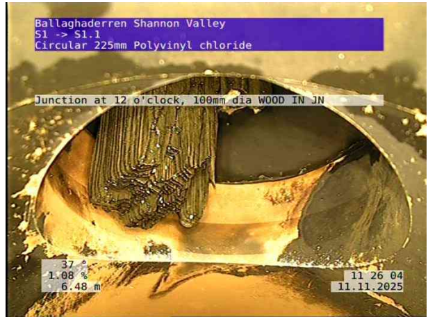
2, 00:01:03, 6.48 m Junction at 12 o'clock, 100mm dia, WOOD IN JN
