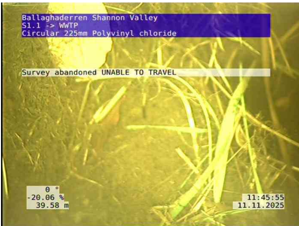
7, 00:11:02, 39.58 m Survey abandoned, UNABLE TO TRAVEL (OUTFALL) (REF CHANGE)
