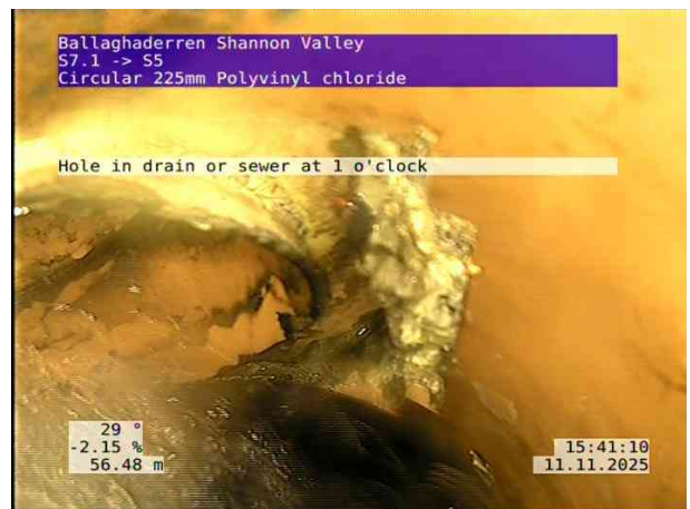
8, 00:06:39, 56.48 m Hole in drain or sewer at 1 o'clock
