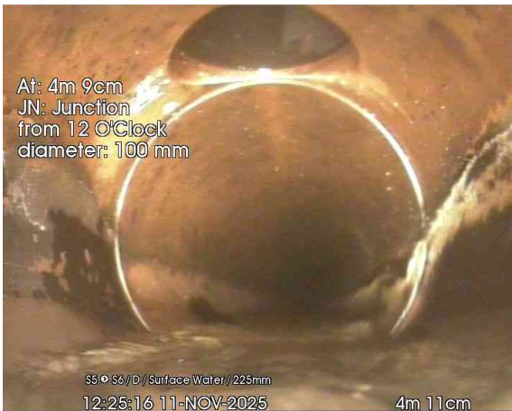
3, 00:00:24, 4.11 m Junction at 12 o'clock, 100mm dia
