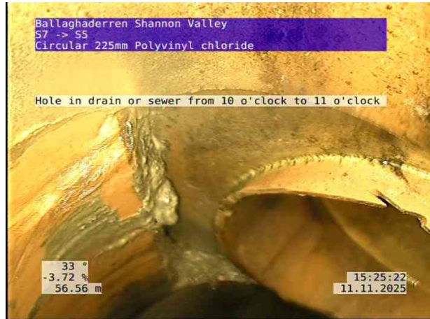
10, 00:06:29, 56.56 m Hole in drain or sewer from 10 o'clock to 11 o'clock
