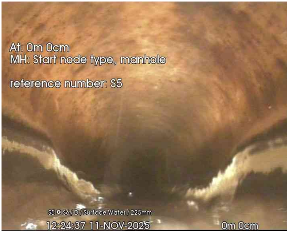
1, 00:00:02, 0.00 m Start node, manhole, reference: S5
