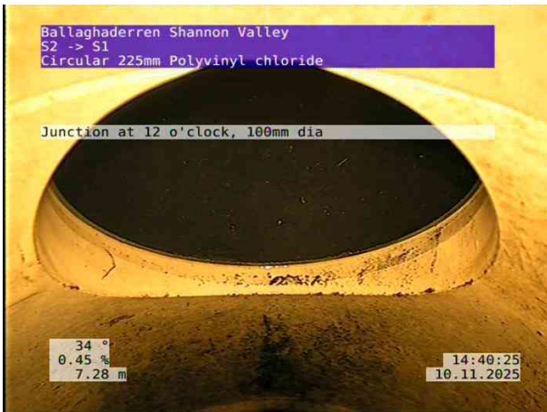
3, 00:01:14, 7.28 m Junction at 12 o'clock, 100mm dia
