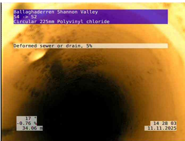
7, 00:04:15, 34.07 m Deformed sewer or drain, 5%
