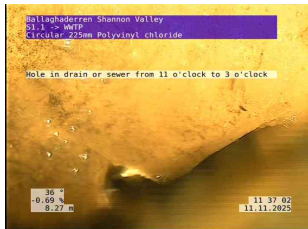
4, 00:02:48, 8.27 m Hole in drain or sewer from 11 o'clock to 3 o'clock
