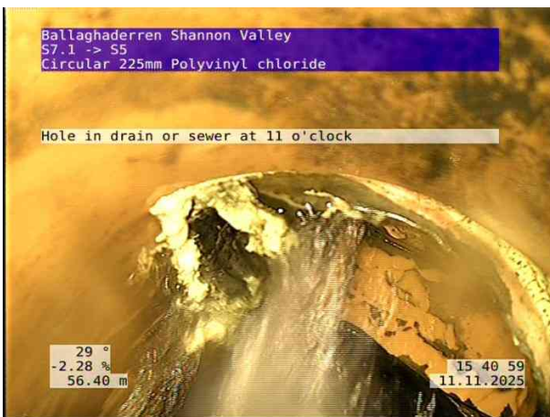
7, 00:06:32, 56.40 m Hole in drain or sewer at 11 o'clock
