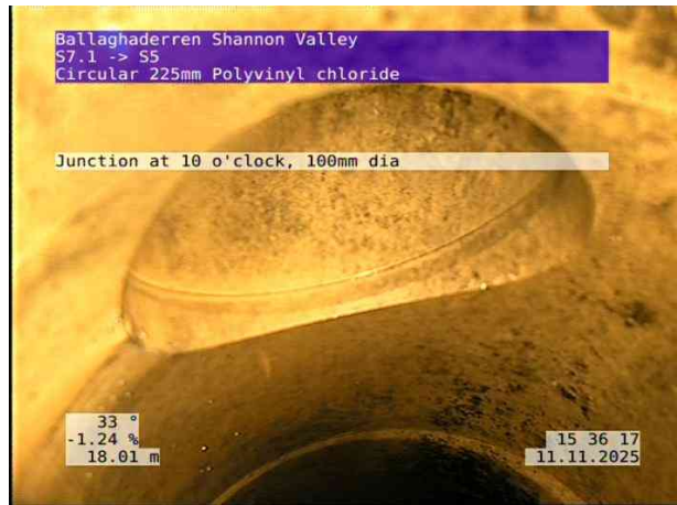
2, 00:02:39, 18.01 m Junction at 10 o'clock, 100mm dia
