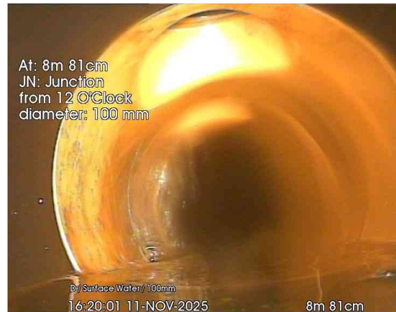
4, 00:00:37, 8.81 m Junction at 12 o'clock, 100mm dia
