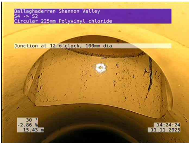
3, 00:01:56, 15.43 m Junction at 12 o'clock, 100mm dia
