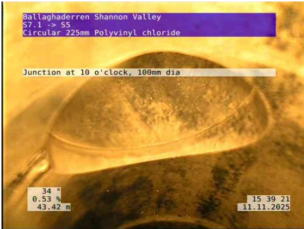
5, 00:05:13, 43.42 m Junction at 10 o'clock, 100mm dia
