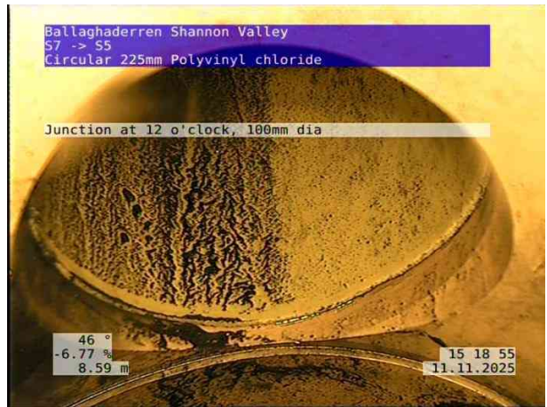
2, 00:01:06, 8.59 m Junction at 12 o'clock, 100mm dia
