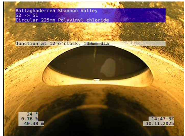
8, 00:07:24, 40.38 m Junction at 12 o'clock, 100mm dia
