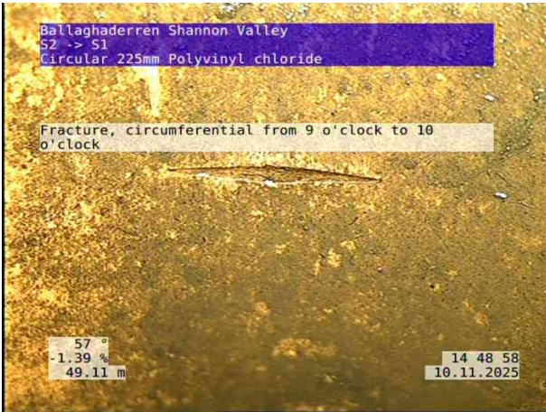
9, 00:08:28, 49.11 m Fracture, circumferential from 9 o'clock to 10 o'clock
