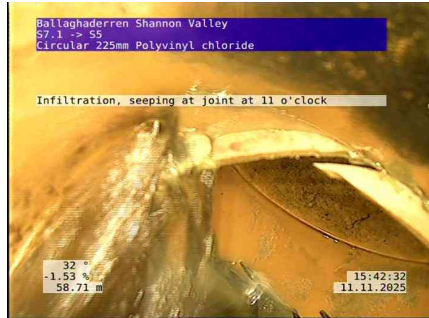
10, 00:07:20, 58.71 m Infiltration, seeping at joint at 11 o'clock
