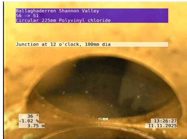
2, 00:00:35, 3.75 m Junction at 12 o'clock, 100mm dia
