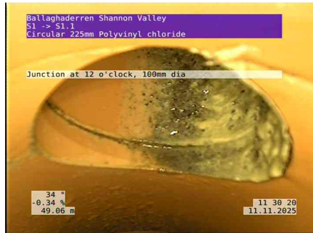
6, 00:04:49, 49.06 m Junction at 12 o'clock, 100mm dia
