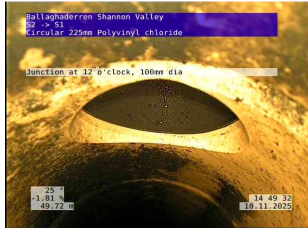
10, 00:08:57, 49.72 m Junction at 12 o'clock, 100mm dia
