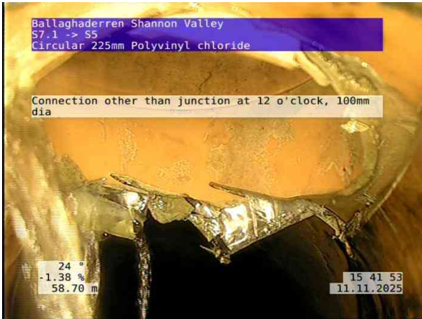
9, 00:07:08, 58.70 m Connection other than junction at 12 o'clock, 100mm dia
