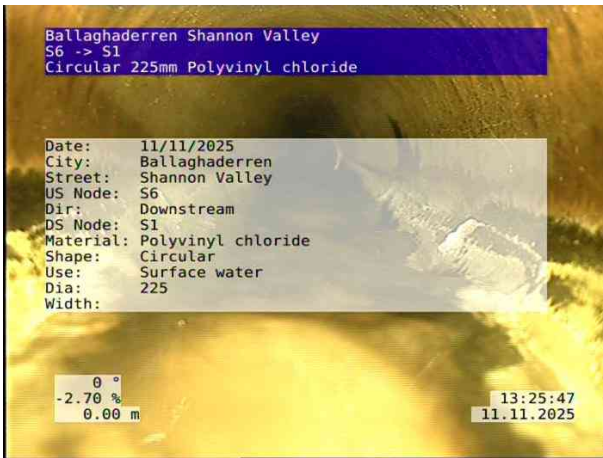
1, 00:00:00, 0.00 m Start node, manhole, reference: S6
