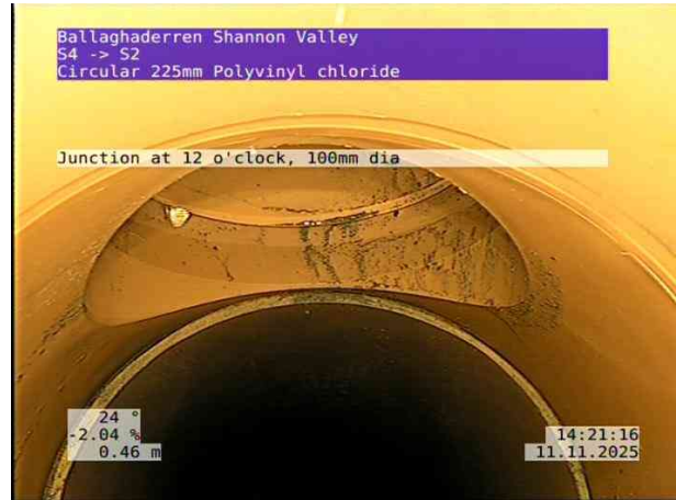
2, 00:00:19, 0.46 m Junction at 12 o'clock, 100mm dia
