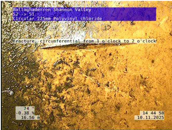
5, 00:04:54, 16.56 m Fracture, circumferential from 1 o'clock to 2 o'clock
