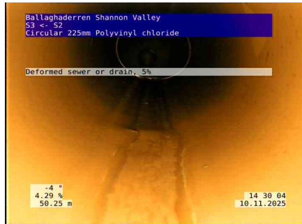
8, 00:05:29, 50.25 m Deformed sewer or drain, 5%
