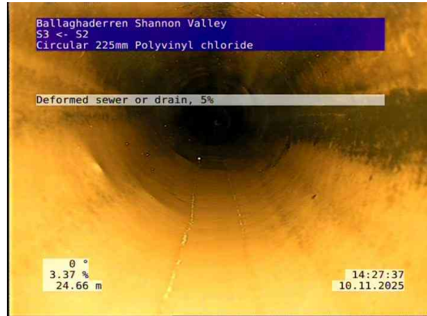
6, 00:03:09, 24.66 m Deformed sewer or drain, 5%
