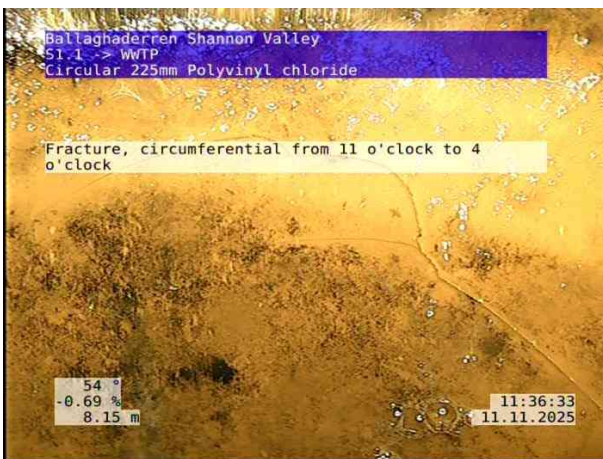
3, 00:02:27, 8.15 m Fracture, circumferential from 11 o'clock to 4 o'clock
