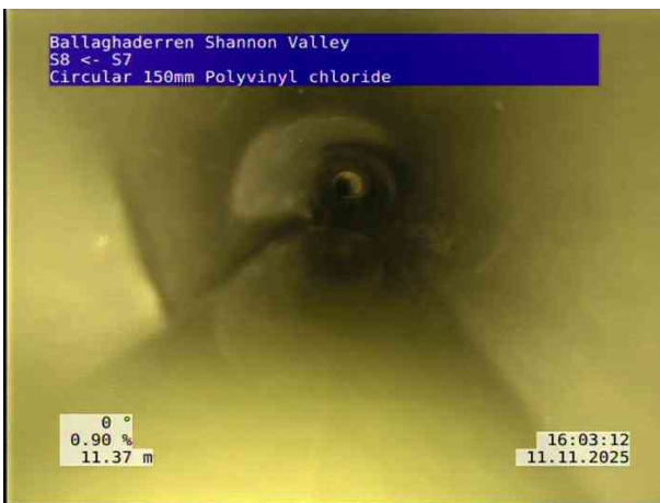
3, 00:02:18, 11.40 m Deformed sewer or drain, 5%
