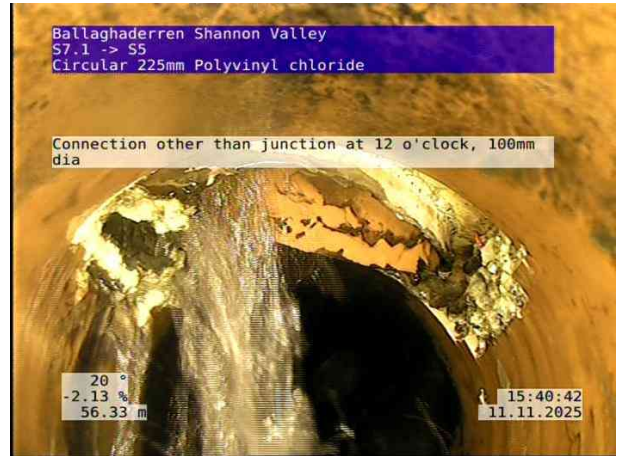
6, 00:06:25, 56.33 m Connection other than junction at 12 o'clock, 100mm dia
