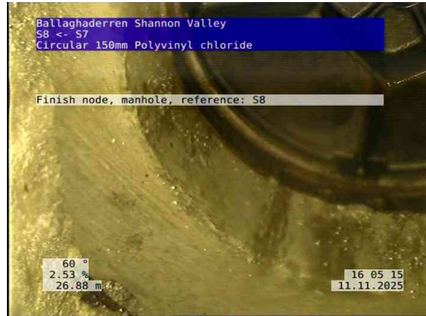
6, 00:04:11, 26.88 m Finish node, manhole, reference: S8
