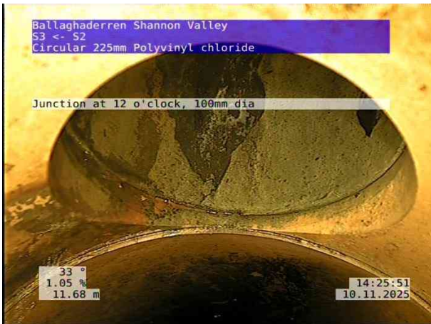
3, 00:01:38, 11.68 m Junction at 12 o'clock, 100mm dia
