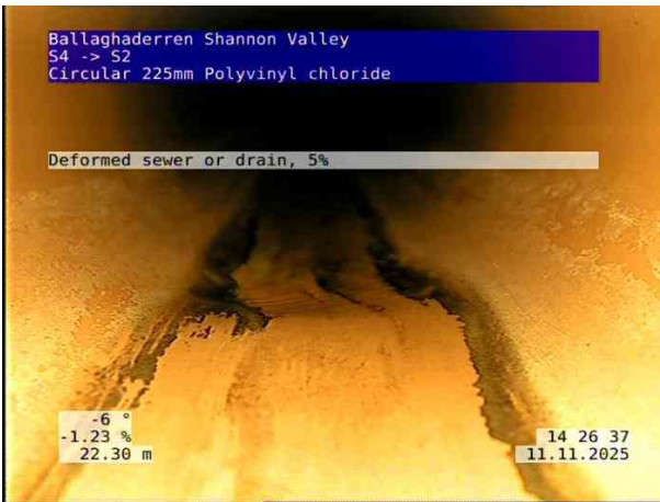
5, 00:02:58, 22.30 m Deformed sewer or drain, 5%
