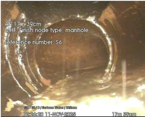
5, 00:01:13, 17.39 m Finish node, manhole, reference: S6
