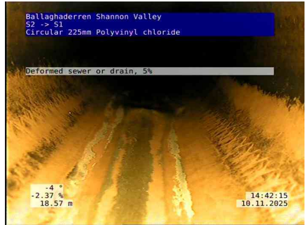
6, 00:02:52, 18.57 m Deformed sewer or drain, 5%
