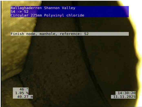
9, 00:06:27, 40.27 m Finish node, manhole, reference: S2
