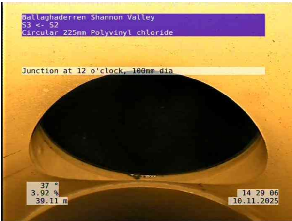
7, 00:04:35, 39.11 m Junction at 12 o'clock, 100mm dia
