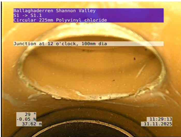
5, 00:03:49, 37.62 m Junction at 12 o'clock, 100mm dia
