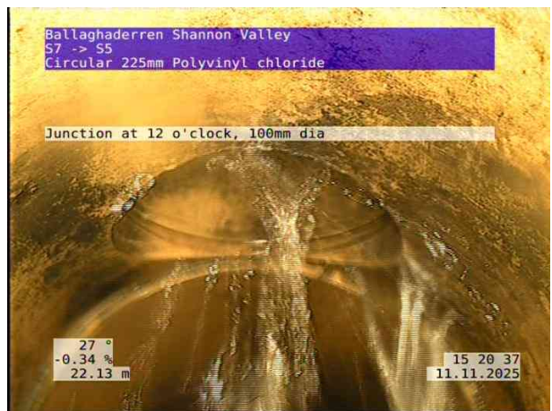
4, 00:02:34, 22.13 m Junction at 12 o'clock, 100mm dia
