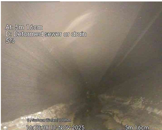
3, 00:00:24, 5.16 m Deformed sewer or drain, 5%
