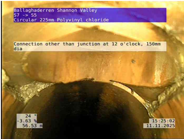
9, 00:06:20, 56.53 m Connection other than junction at 12 o'clock, 150mm dia
